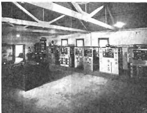
The transmitting studio of VK3ME installed at Braybrook, near Melbourne, Victoria, Australia. This short wave transmitter was designed and manufactured in Australia by Amalgamated Wireless (A'sia) Ltd.
